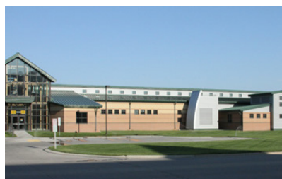
North Dakota State Univ., Ag. Service Ctr. Greenhouse Complex, BLP-3 Bldg.
