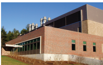
Tufts New England Reg. Biosafety, New Lab Bldg. & APVs
