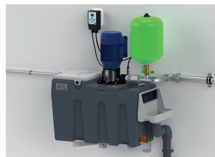
DPVCI installed in a DP HUV1 Eco Break.
